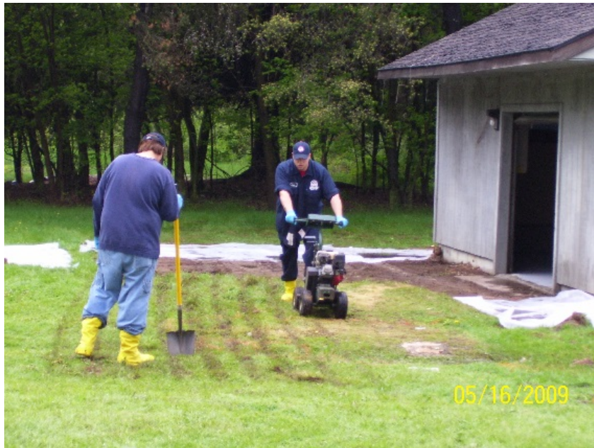
Photograph 9-16 View of a soil/sod cutting operation
