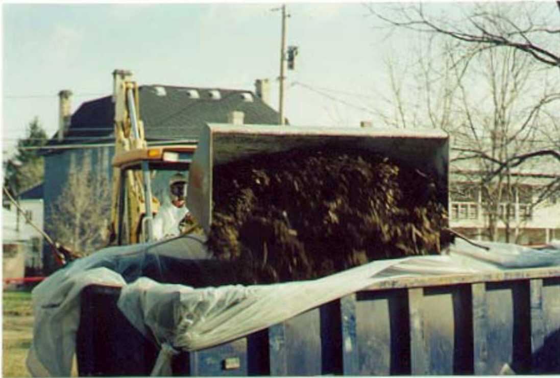
Photograph 9-19 View of mercury-contaminated soil being staged into a plastic-lined rolloff box
