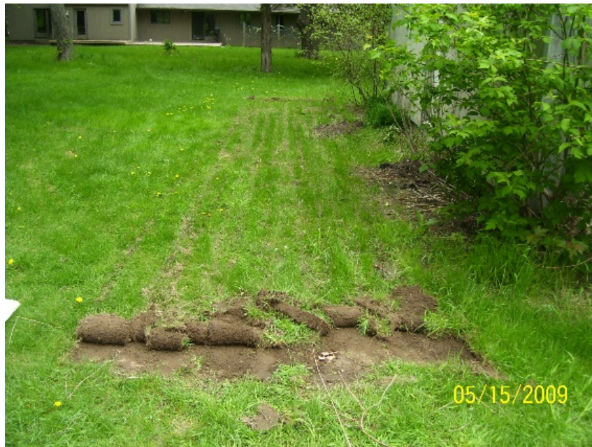
Photograph 9-17 View of a soil/sod cutting operation
