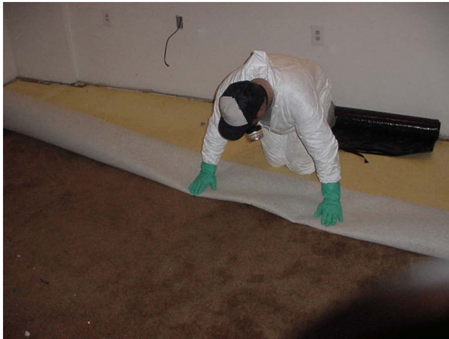
Photograph 9-9 View of carpet removal
