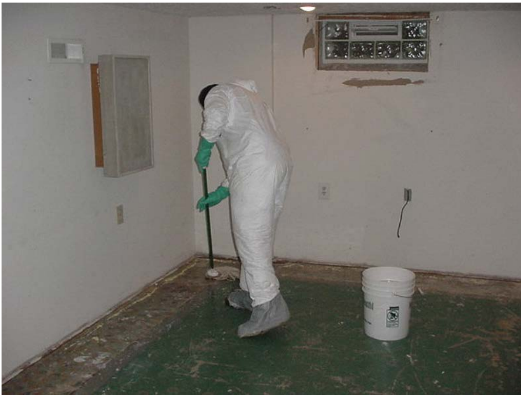
Photograph 9-4 Mopping floors with mercury treatment solution
