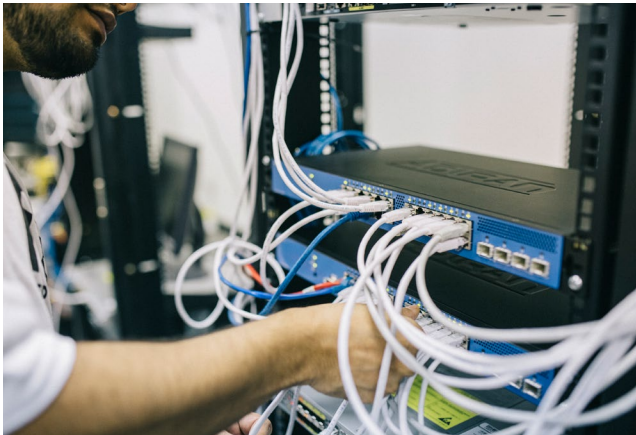
Work-tech student working on a telecommunications project.
