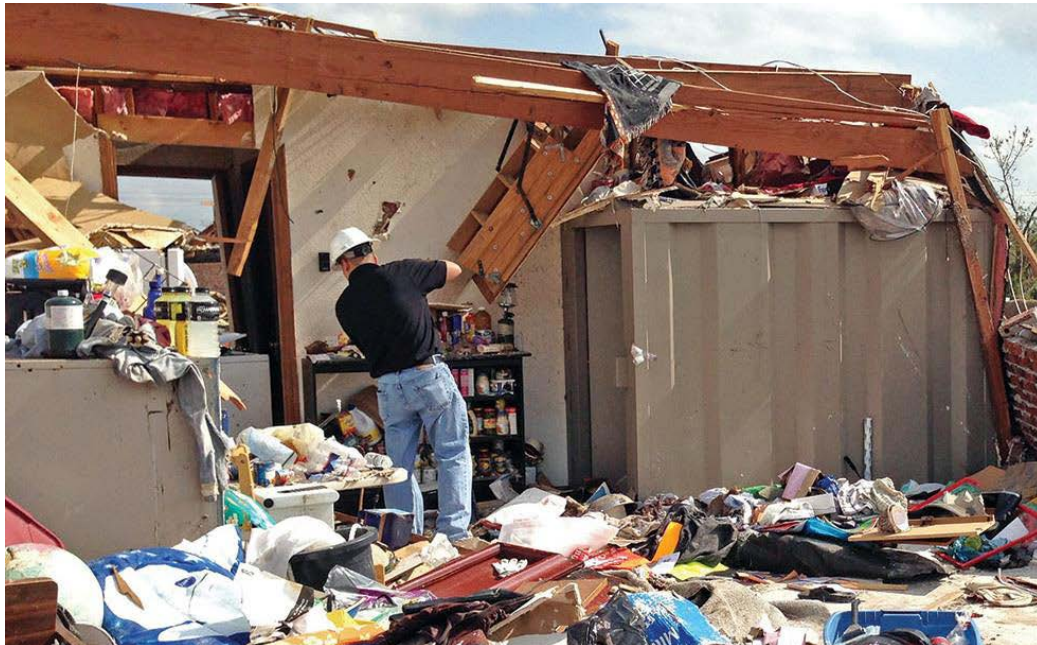
Figure 6. A local building code inspector inspects an above-ground shelter that performed well in a heavily damaged area
