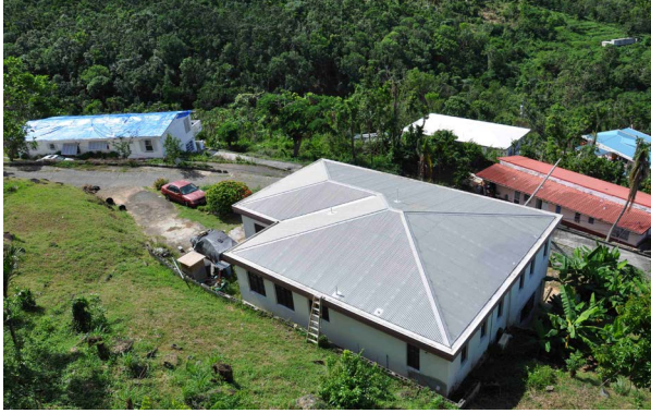
Figure 1. USVI home built using 1994 code
