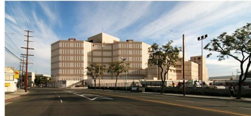
Twin Towers Correctional Facility ~ 3500
