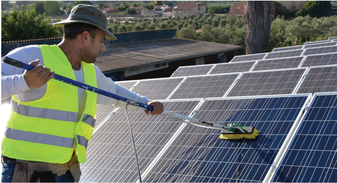
A person wearing a yellow safety vest cleans a rooftop solar panel..
