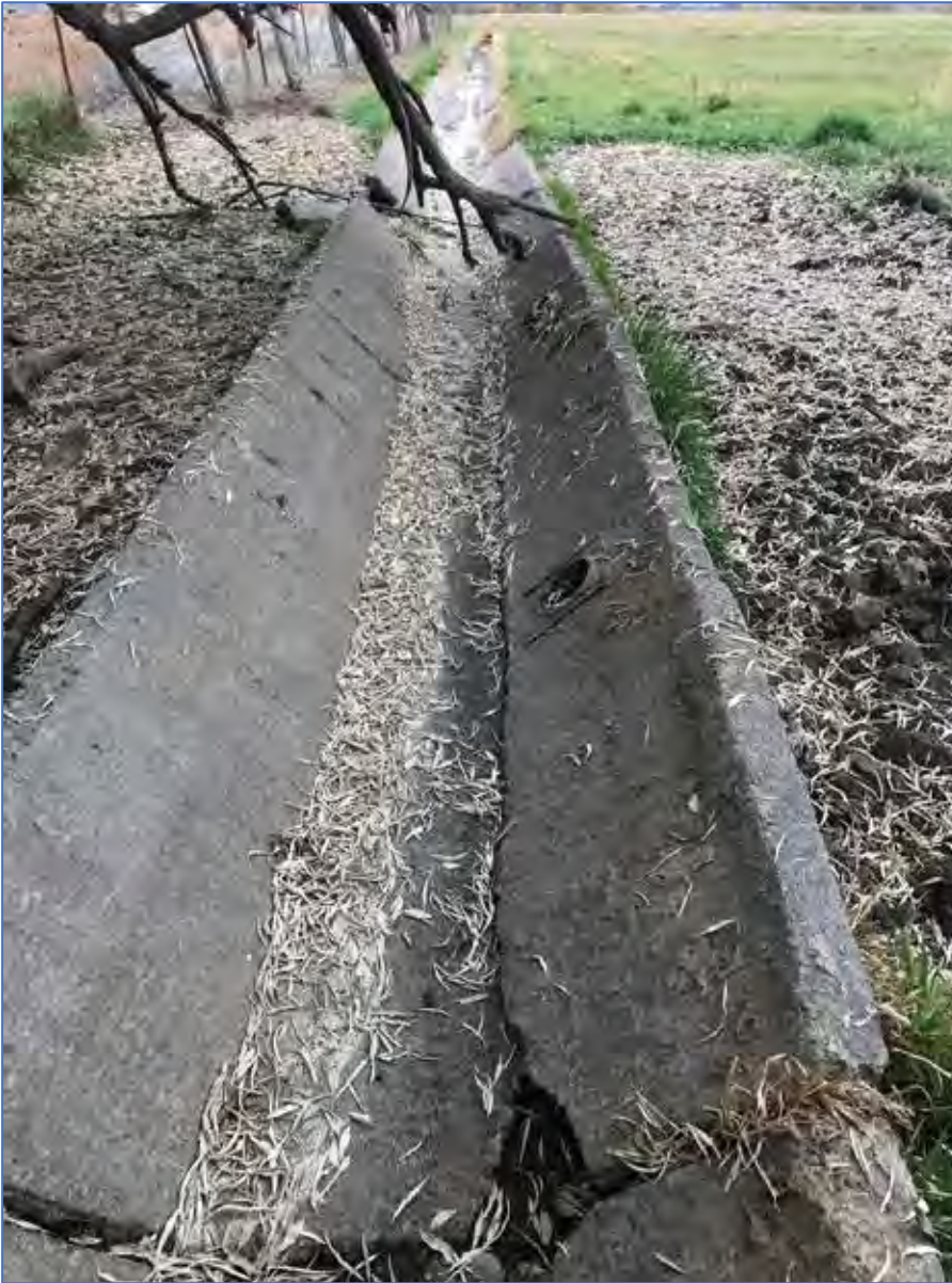
Photo 11 View east from Photo Point 7, ditch D3.
