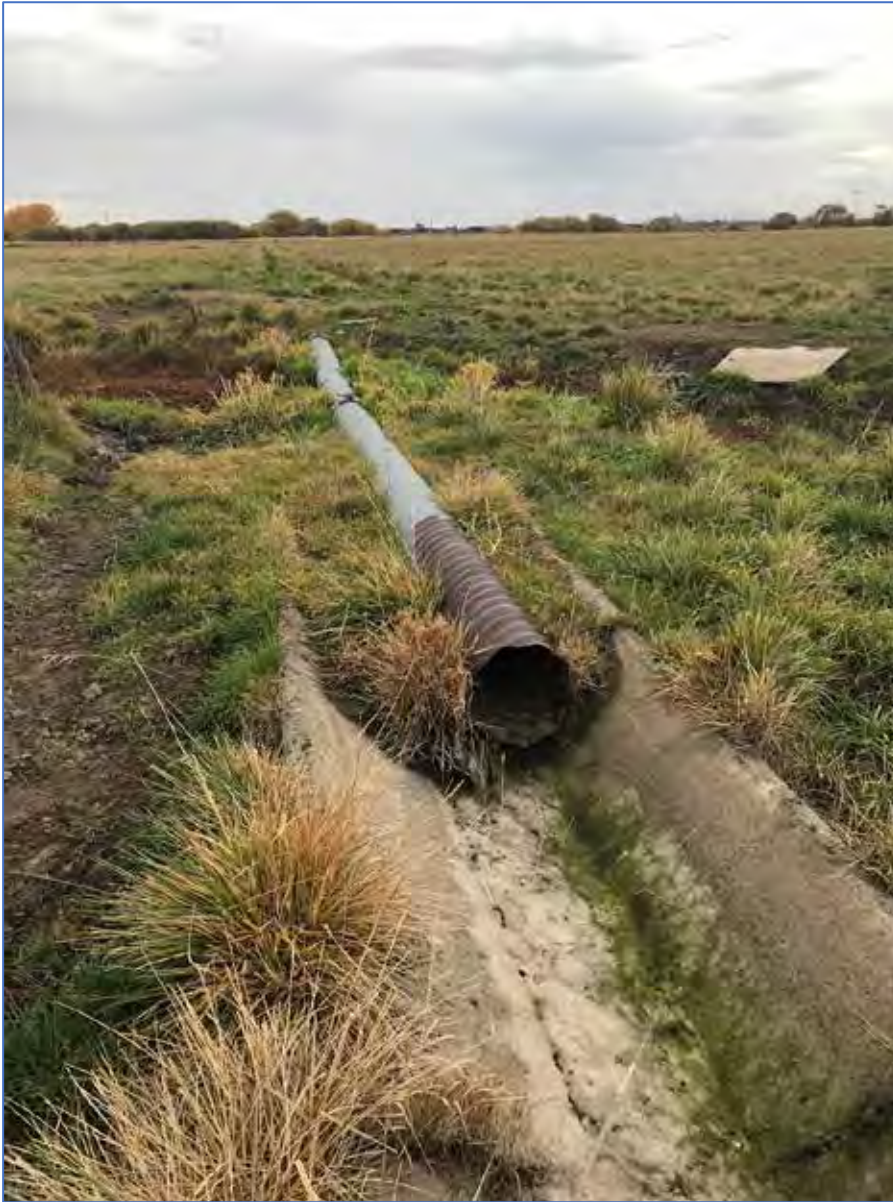
Photo 12 View east from Photo Point 8, ditch D3 crossing of ditch D1.
