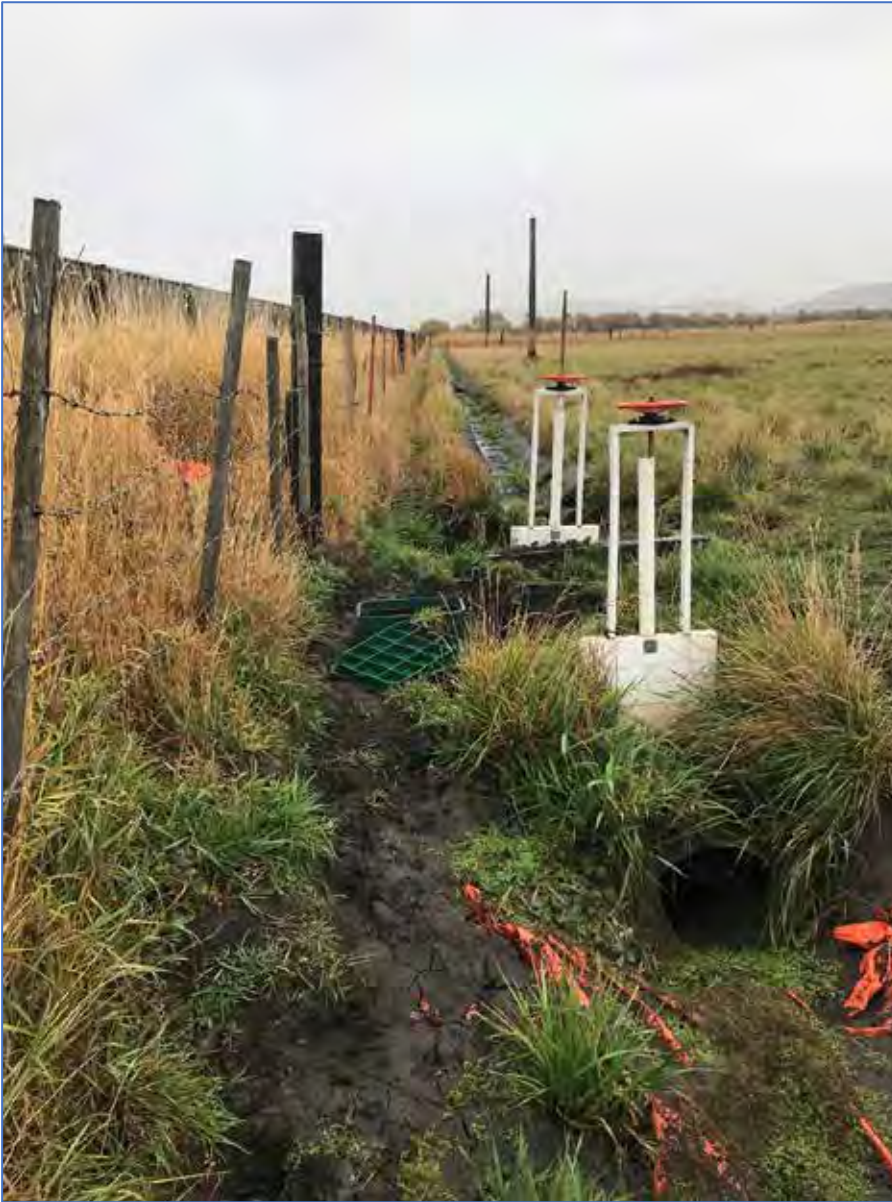
Photo 23 View east from Photo Point 18, water control structure in ditch D7.
