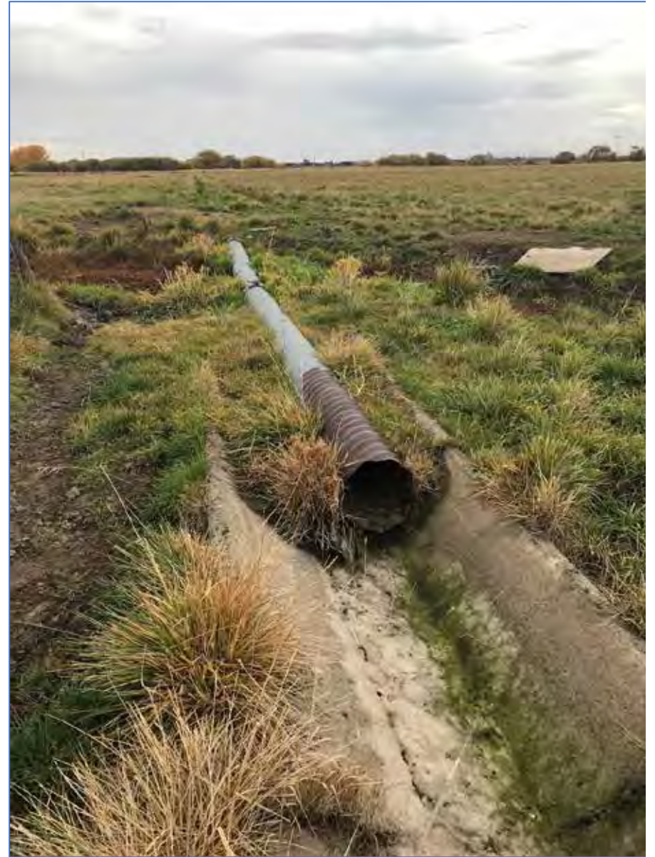
Photo 12 View east from Photo Point 8, ditch D3 crossing of ditch D1.
