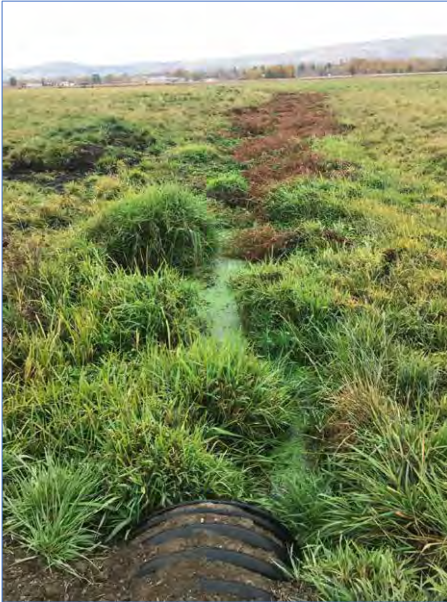
Photo 17 View south from Photo Point 13, ditch D1.
