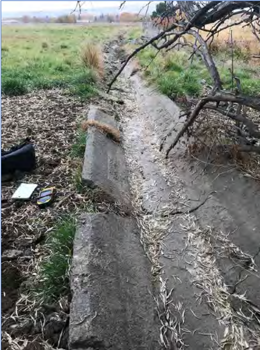
Photo 10 View south from Photo Point 7, ditch D3.
