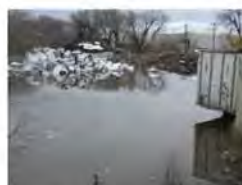
Water surrounds the large home appliance drop-off area
