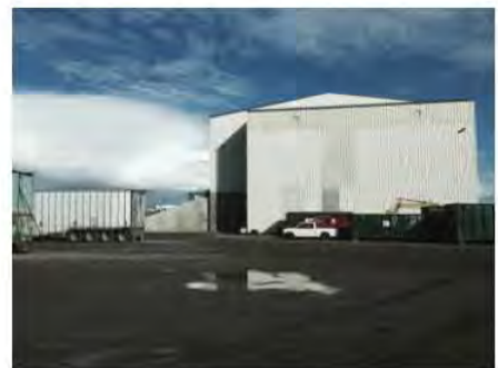
Side of the Transfer Building (for garbage)
