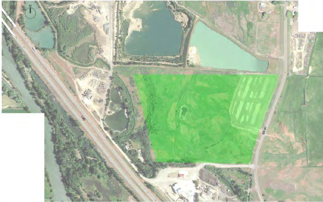
CEMENT PLANT SITE
