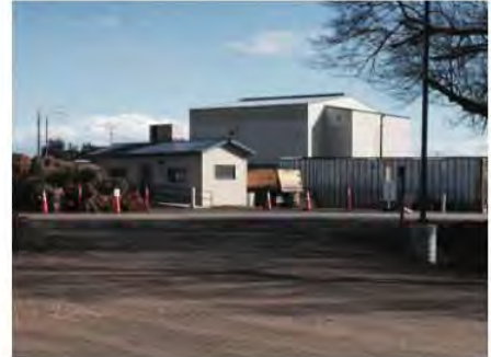
Scalehouse at entrance to transfer station
